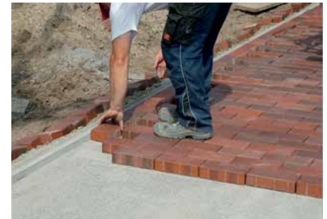
Fig. 5-11: Laying of clinker pavers by hand
