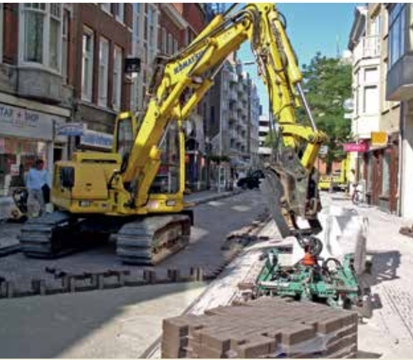
Machine laying of clinker pavers, Den Haag, the Netherlands
